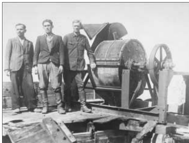
Wartime photo showing Heinrich Chamaides, Moische Korn and David Manusevich next to a ball mill used for road construction.
